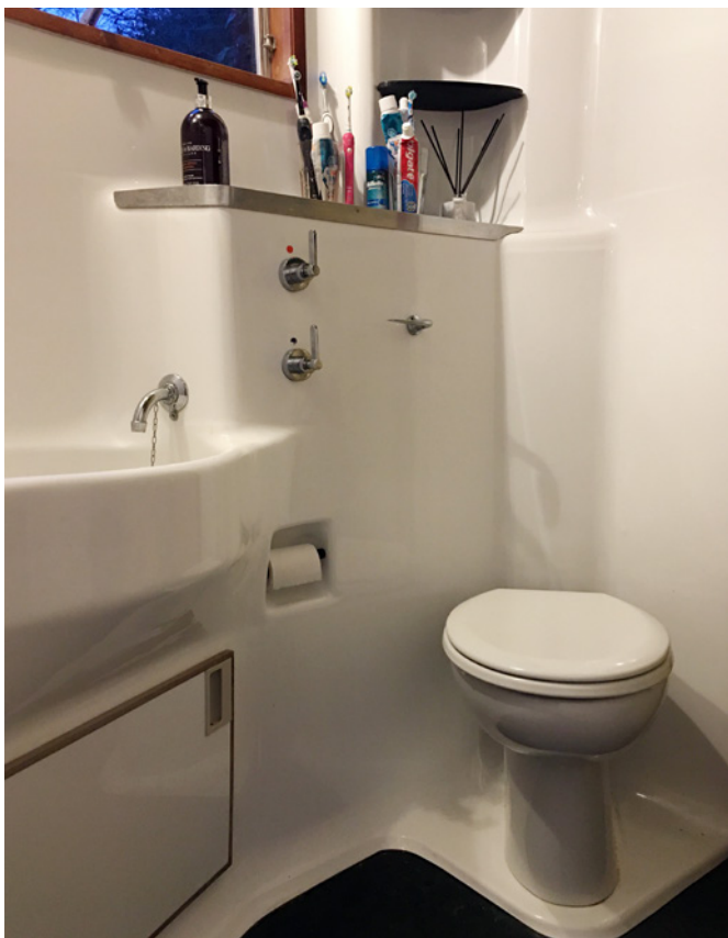
13 Intact ICI prototype acrylic bathroom, Hartford, England. © R. Loader, November 2021
