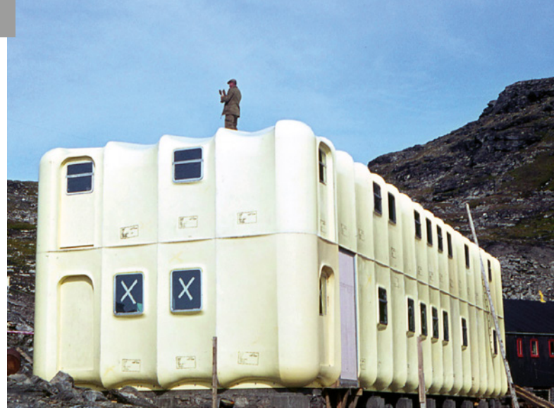
01 The Biological Research Laboratory at Signy Island, Antarctica, nearing completion in April 1964. Double curvature GRP panels produced by Mickleover Transport. © F. Topcliffe, 26 February 1964. Reproduced courtesy of the British Antarctic Survey Archives Service. Archives ref. 2006/2.1
