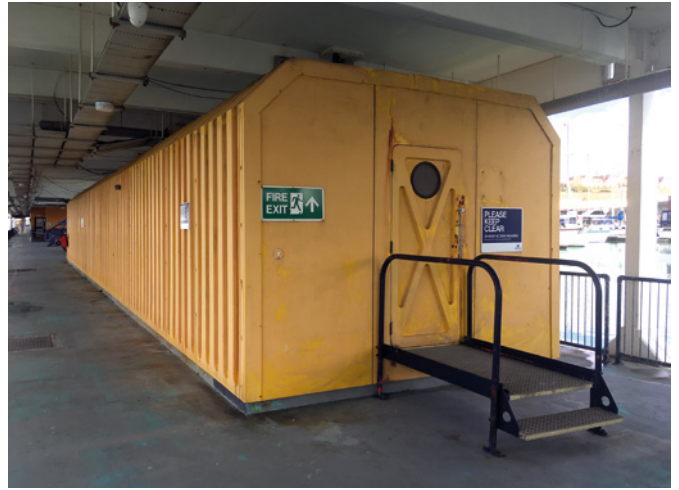
10 Building for Yachtsmen's Showers and Lavatories at Brighton Marina. © R. Loader, October 2019
