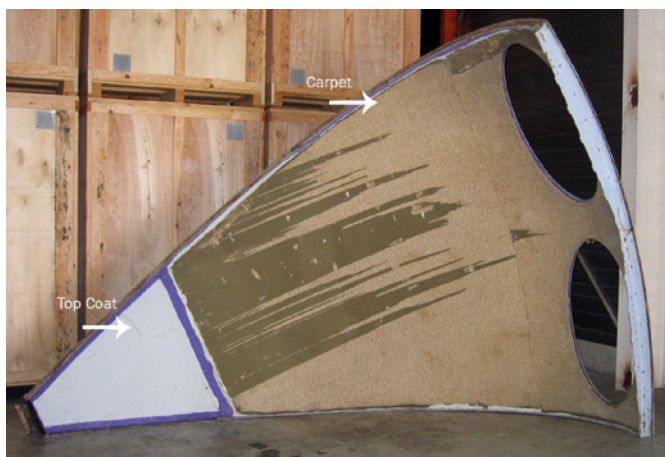
03 Interior of the Futuro house, 2007. Arrows show the layer of top coat with a grayish color on top of purple primer and the presence of a synthetic carpet at the lower part of the segment. © E. Stamatopoulou, 2008
