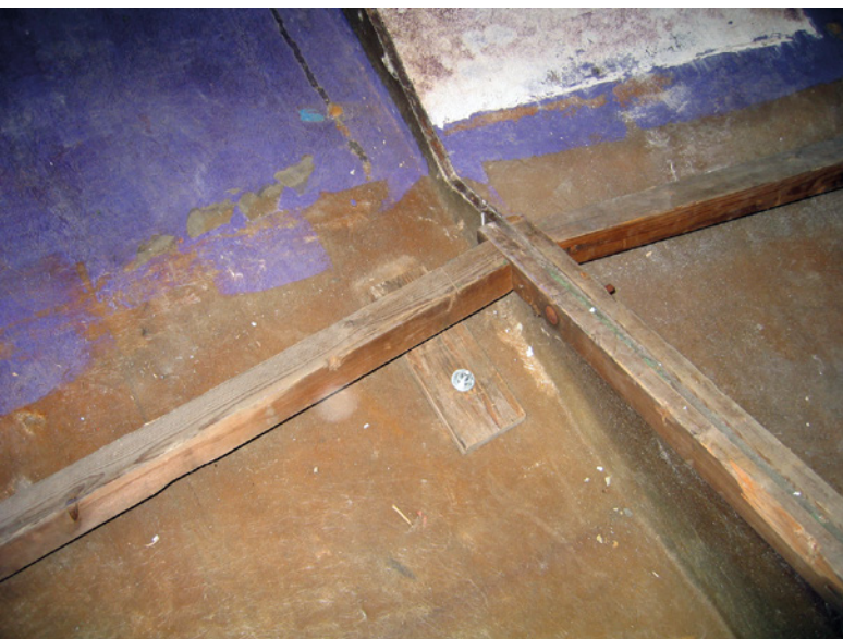
01 Wooden reinforcement of the lower elements of the building, covered with the characteristic purple and grayish topcoat. © E. Stamatopoulou, 2008
