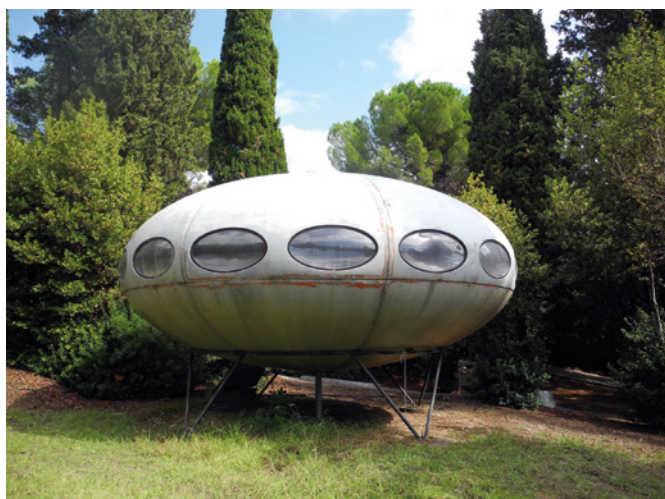
06 The Futuro house installed in Limni, Corfu, in its current condition. © E. Stamatopoulou, 2019
