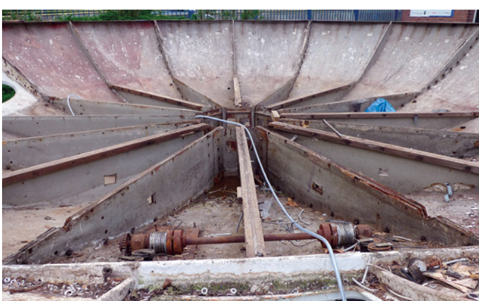
15 Support structure of the Finnish Futuro. © P. Voigt, 2016
