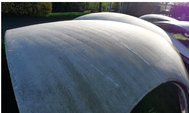
13 Cutting and orientation of the PUR insulation in the sandwich visible in sidelight. © P. Voigt, 2016
