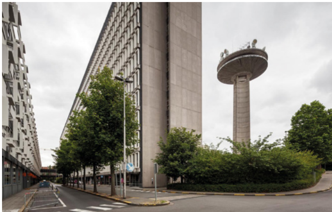
05 View of the BRT Center. © N. Serneels
