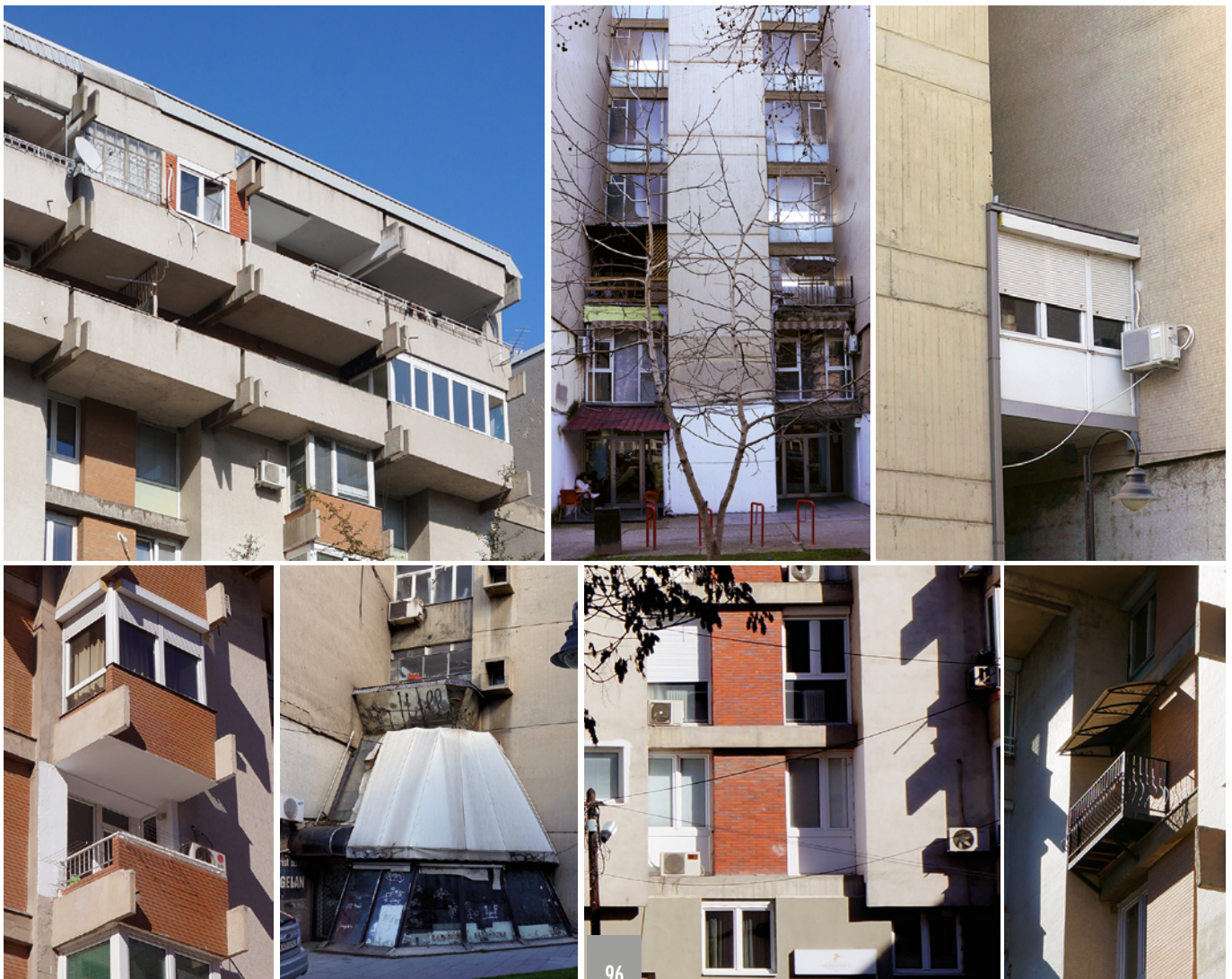
09 Alterations carried out by the dwellers, including sloped roof cover, enclosing parts of the terraces, adding new balconies, turning bay windows into balconies and other changes and additions to the façades © Vlatko P. Korobar, 2023.
