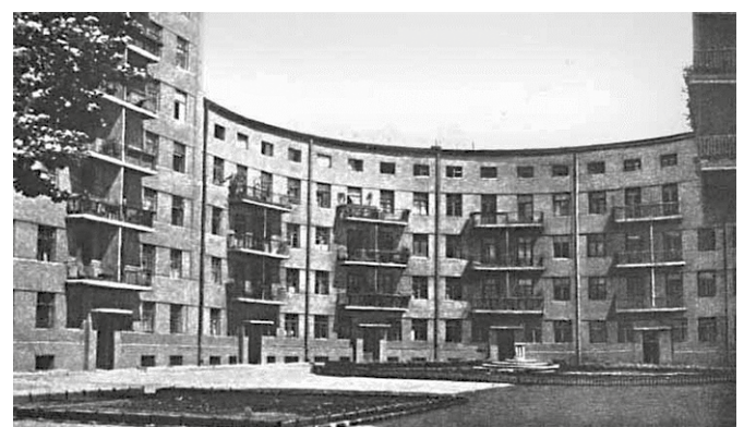
07 Komunar (Communard) residential house, 1929-1930, arch. A. V. Linetskyj and V. I. Bogomolov. © prof. A. Bouryak's personal archives.
