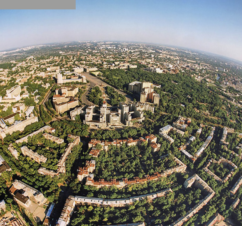
01 Aerial view of the Freedom Square complex in Kharkiv. © V. Bysov, 2002.
