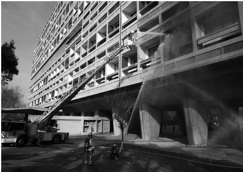
Figure 1. Le Corbusier , Unité d'habitation , Marseille (1945-1952), fire on February 9, 2012.
