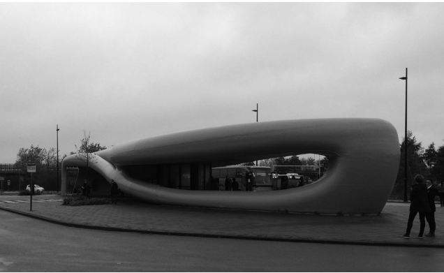
05 Nio Architects, bus station, Hoofddorp, The Netherlands, 2003. The polyester skin was made on site by Poly Products. © Wessel de Jonge.
