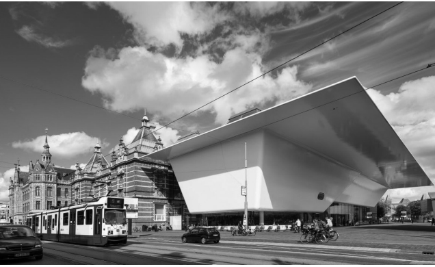
03 Benthem Crowwel Architekten, Stedelijk Museum extension, Amsterdam, The Netherlands, 2014. It features an innovative synthetic skin that is almost seamless. © Janne Linders.
