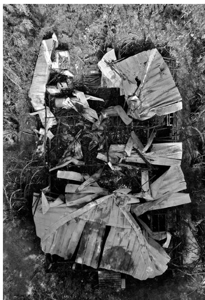
01 Casa Klumb, aerial fire detail. © Javier Olmeda, 2020..
