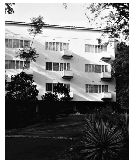
01 Front, (south) elevation, Delamare Flats. © Dennis Sharp Archive.
