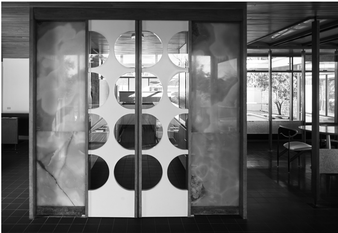
07 Iwan Iwanoff, Paganin House, Perth, Australia, 1965, Paganin House Entry foyer looking towards the kitchen with Laminex and glass sliding doors and translucent marble wall panels, all reproduced in the rebuilt house. © Photo Robert Frith/Acorn Photo.
