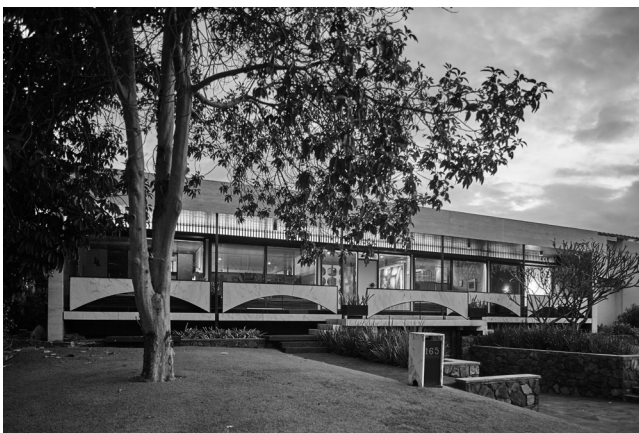
02 Iwan Iwanoff, Paganin House, Perth, Australia, 1965, Paganin House front facade photographed in 2005 prior to the fire during the previous ownership of the house, illustrating the use of white marble on the verandah fascia and balustrade and the extensive use of Western Australian Jarrah hardwood timber on the verandah soffit and the front (North-facing) facade window wall. © Photo Robert Frith/Acorn Photo.
