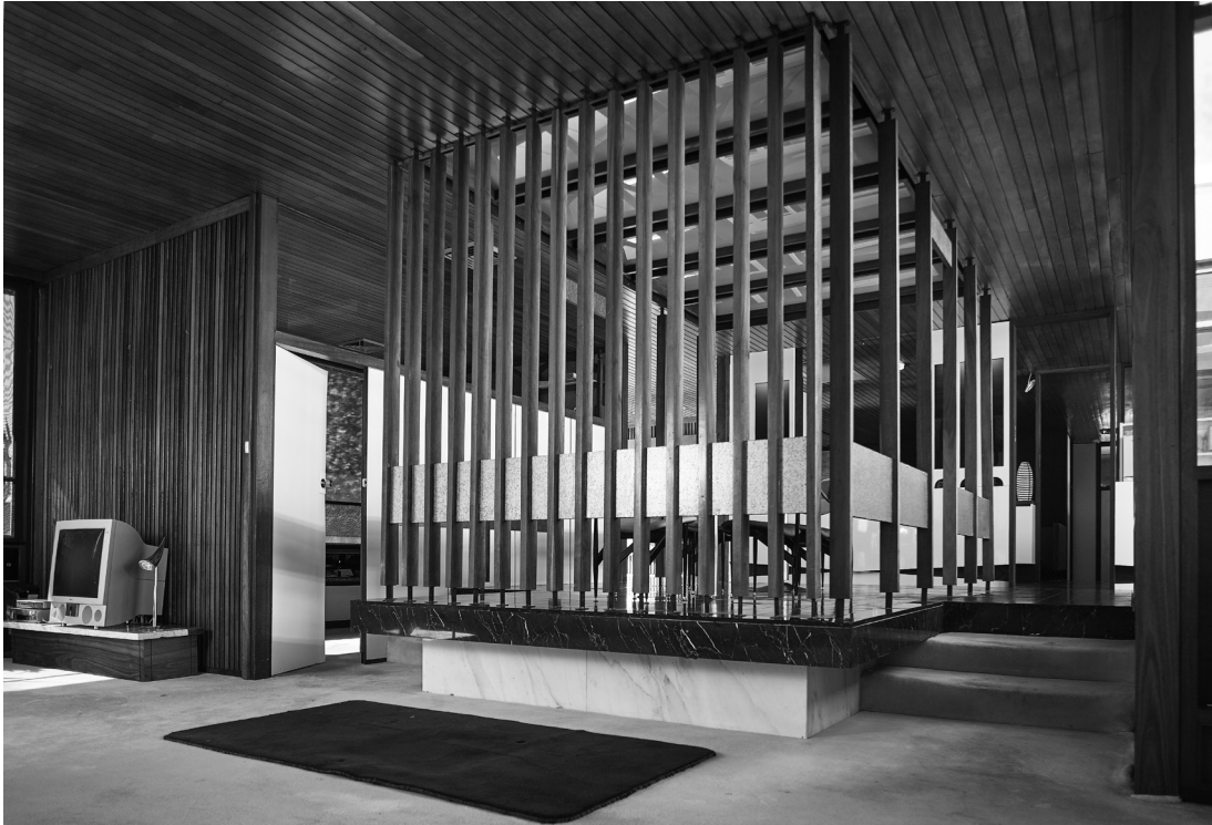
08 Iwan Iwanoff, Paganin House, Perth, Australia, 1965, Paganin House Dining area with timber screen, the main Jarrah timber ceiling and wall paneling, all reproduced in the rebuilt house. The barrel-vaulted white Perspex lighting diffuser ceiling over the Dining area was also replicated in the rebuilt house. Photographed in 2005 prior to the fire during the previous ownership of the house. © Photo Robert Frith/Acorn Photo.
