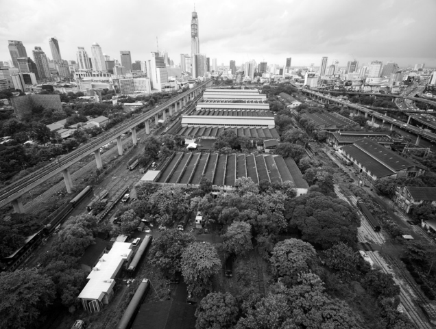
01 Makkasan Factory land, bird eyes view. © Survey and Inventory of Valuable Buildings Worthy of Preservation in Makkasan Factory District, 2017.
