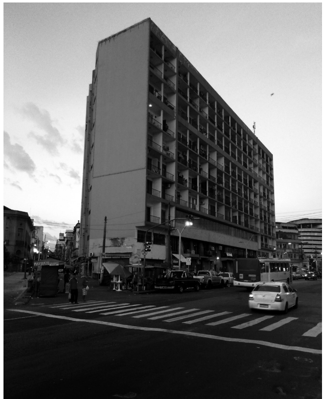
07 Paulo Antunes Ribeiro, Hotel Amazonas , Manaus, Brazil, 1947-1952. Current state of conservation, 2018. © Photographed by Ricardo Paiva.
