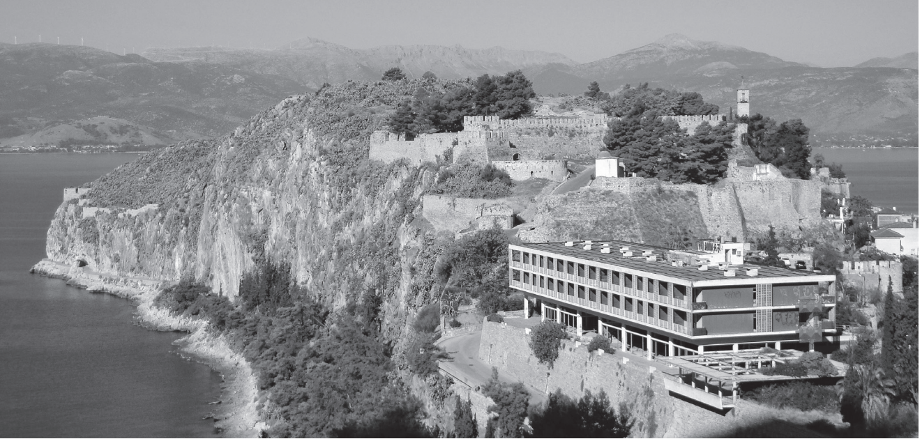
03 Yannis Triantafyllidis, Akronafplia Xenia Hotel, Nafplio, Greece, 1961. Currently abandoned. © Stavros Alifragkis, September 2012.
