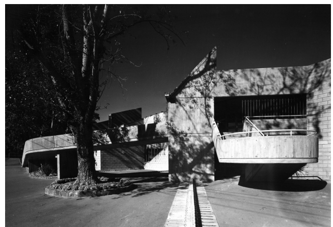
07 Borland & Jackson Architects, Harold Holt Memorial Swimming Centre, Malvern, Victoria, 1969. © Courtesy Doug Evans.
