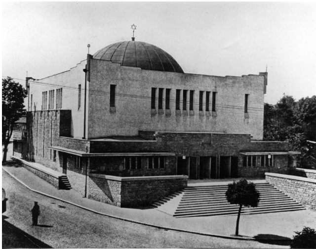
01 Peter Behrens, the New Synagogue, Žilina, Slovakia, 1931. View of the exterior. © HÚ SAV Bratislava.
