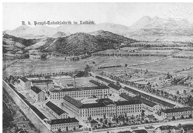
03 Tobačna Tovarna [Tobacco Factory], Ljubljana, 1873. Typical industrial architecture of the 2 nd half of the 19 th century, situated on the city outskirts, next to the railway. Built in a brick external structure, with an internal system of cast iron columns and beams. © Sonja Ilko.
