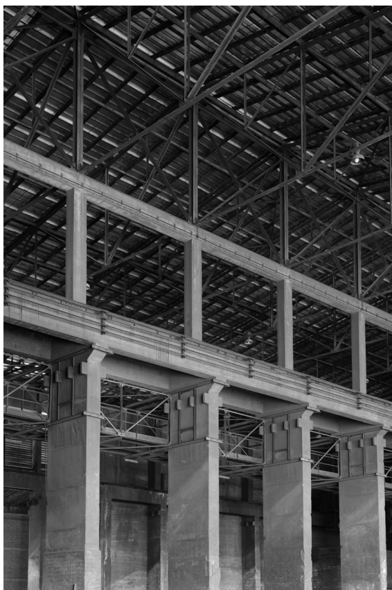
06 Building for bauxite processing, Alumina and aluminum plant, Kidričevo, 1943-1954. © Miran Kambič.
