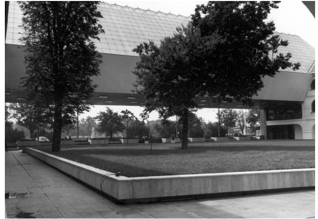
06 Vladimír Dedeček, Slovak National Gallery, Bratislava, Slovakia, 1967-1979. View from the courtyard to the glass roof of the exhibition block. © Archive of Department of Architecture HÚ SAV.
