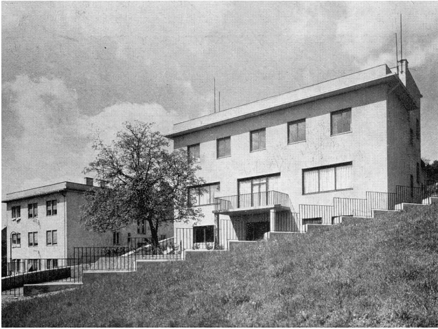
01 Friedrich Weinwurm and Ignác Vécsei, Villa Lengyel, Bratislava, Slovakia, 1929. View of the villa and apartment block by the same authors. © Archive of Architecture oA HU SAV.
