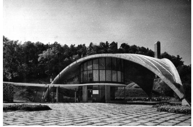
02 István Bérces, Miklós Gnädig, Béla Szittyá, Old port, Tihany, Hungary, 1962. The concrete shell structure. © 1960s, IPARTERV photo archive, No 6051.
