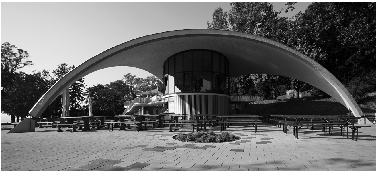
05 László Földes, András Farkas, Péter Sugár, Old port, Tihany, Hungary, 2015. Information centre and buffet under the reconstructed concrete shell structure. © Tamás Bujnovszky, 2015.
