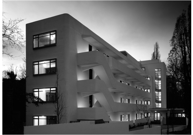
07 Wells Coates, Lawn Road Flats (The Isokon), London, UK, 1933-34. Restoration completed by Avanti Architects. © Nicholas Kane, courtesy Avanti Architects, 2005.
