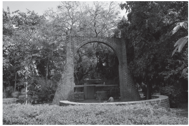
04 Louis Kahn, Indian Institute of Management in Ahmedabad, India, 1962-1974. Experimental arch built to demonstrate the construction under Kahn's supervision in 1970. © SNK, 2015.
