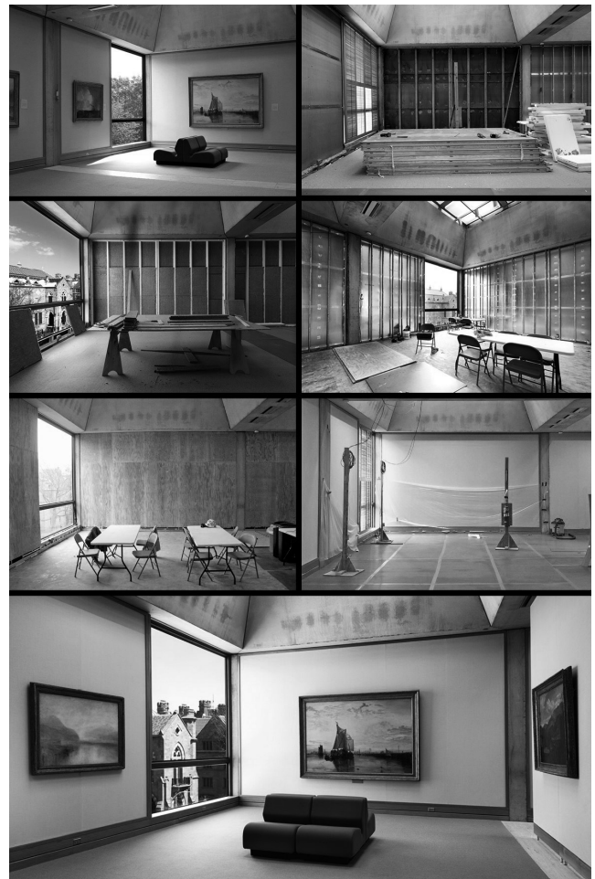
09 Louis Kahn, Yale Center for British Art, New Haven, USA, 1966-1977. Fourth floor "Turner Bay" displaying the exterior wall sequence that was typical throughout the project spaces. Top to bottom, left to right: 1) pre-conservation, 2) exterior panels, 3) insulation, 4) air barrier, 5) substrate, 6) finishes, 7) post-conservation. © 1) Yale Center for British Art, Richard Caspole, 2007, 2-4) 2015, 7) 2016, 5-6) Knight Architecture LLC, Daphne Kalomiris, 2015.
