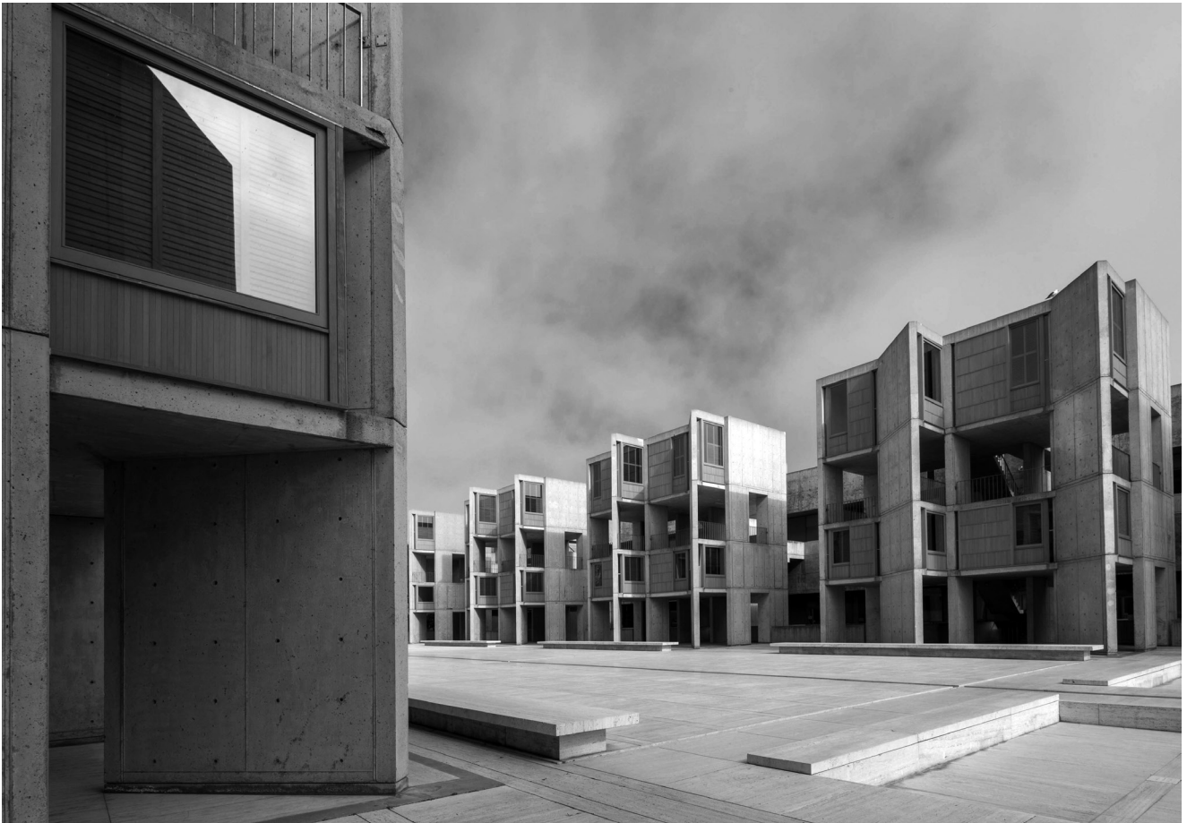
10 Louis Kahn, Salk Institute, La Jolla, California, USA, 1959-1965. Overall view, looking southeast across the plaza, following completion of project. © Elizabeth Daniels, 2017.
