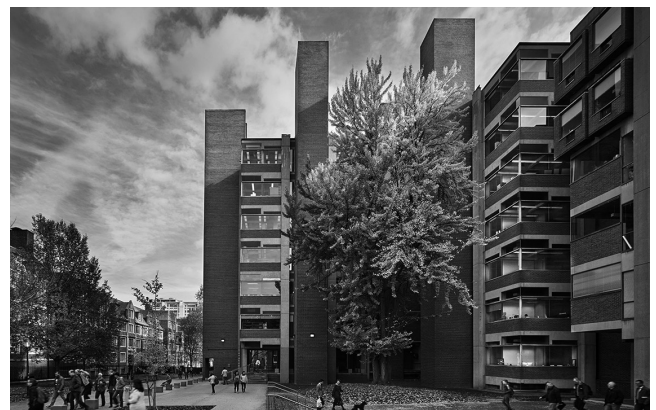
17 Louis Kahn, Richards Bio-Medical Research Laboratories, University of Pennsylvania, Philadelphia, USA, 1957-1961. Exterior from West. © Halkin Mason, 2015.
