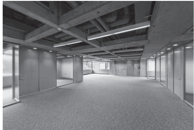
10 Louis Kahn, Richards Bio-Medical Research Laboratories, University of Pennsylvania, Philadelphia, USA, 1957-1961. Completed 6 th floor Tower D workspace prior to furnishing, showing full height glass and wood partitions offset from grid with infill ceiling. © Jeff Goldberg, ESTO, 2015.
