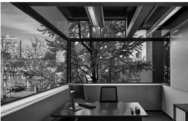
16 Louis Kahn, Richards Bio-Medical Research Laboratories, University of Pennsylvania, Philadelphia, USA, 1957-1961. Typical renovated corner office showing knee-wall enclosure and interior glazing along offset line. © Halkin Mason, 2015.
