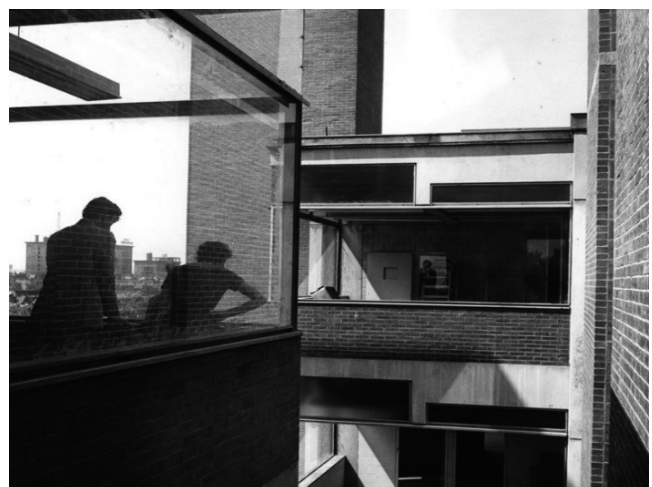
04 Louis Kahn, Richards Laboratories, Philadelphia, USA, 1957-1961. View between two towers showing stainless steel glazing frames. © Mildred Schmeitz Photograph, University of Pennsylvania Architectural Archives, 1961.
