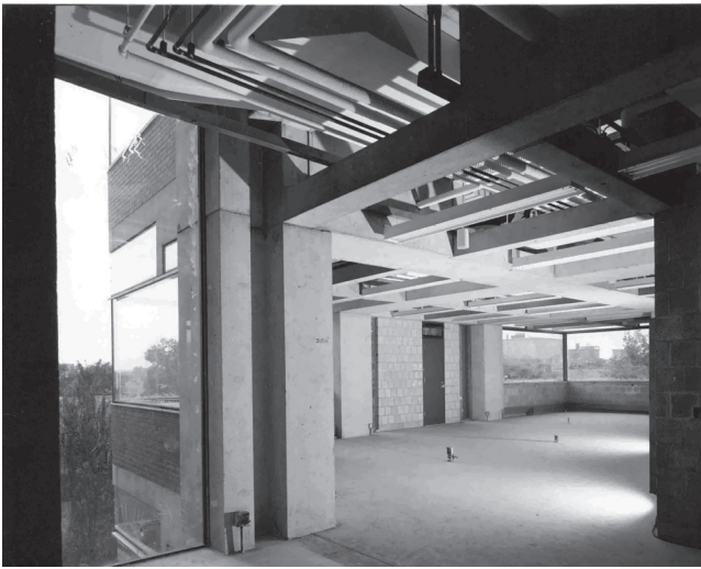
07 Louis Kahn, Richards Bio-Medical Research Laboratories, University of Pennsylvania, Philadelphia, USA, 1957-1961. Interior construction showing routing of systems. © University of Pennsylvania Architectural Archives, 1961.
