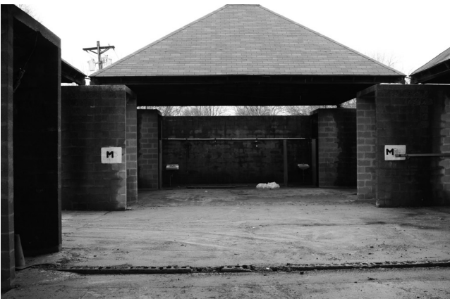
04 Louis Kahn, Trenton Bath House, Ewing, New Jersey, USA, 1955. View of Bath House during construction with removed demising walls. © Mills + Schnoering Architects, LLC, Michael J. Mills, FAIA, 2010.
