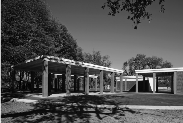
07 Louis Kahn, Day Camp Pavilions, Ewing, New Jersey, USA, 1957. Day Camp Pavilions after restoration. © Brian Rose, 2010.
