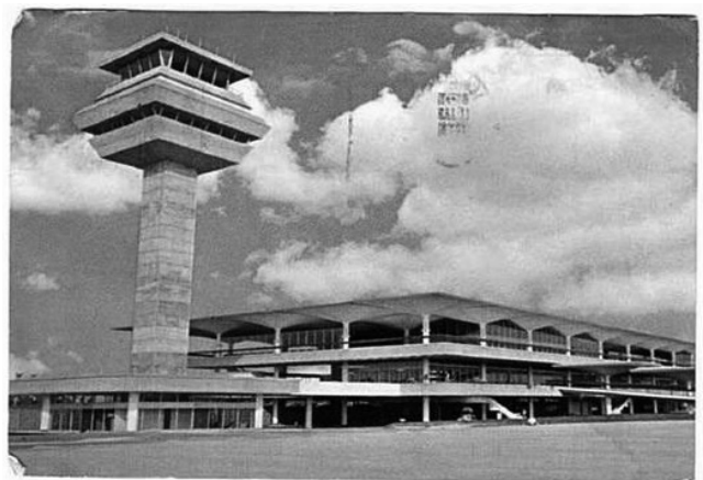
05 Kington Loo of BEP, Kuala Lumpur International Airport, Subang, Malaysia, 1965. With a hyperbolic paraboloid concrete roof and the longest runway in Southeast Asia at the time of its construction, the airport was as one of the most modern airports in the region in the 1960s. © National Archive, 1960s.
