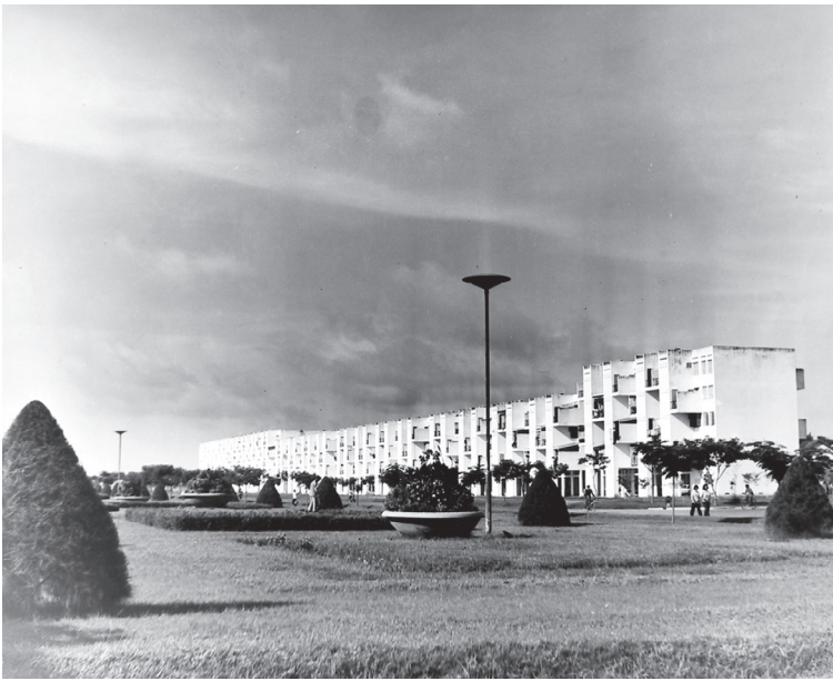
04 Lu Ban Hap, White Building, Phnom Penh, Cambodia, 1963. View from the garden in front of the building. © Vann Molyvann Private Collection.
