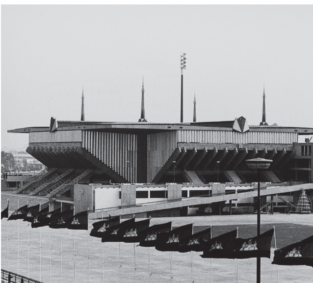
06 Vann Molyvann, Indoor Stadium, Phnom Penh, Cambodia, 1960s. The outside view of the main building of the Olympic National Sports Complex. © Vann Molyvann Private Collection.
