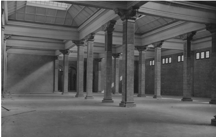
01 Manuel Casas and Manuel Puig, Decorative and Industrial Arts Palace, Barcelona, Spain, 1929. Interior view. Under construction. © AFB, Arxiu Fotogràfic de Barcelona , February 14, 1929.
