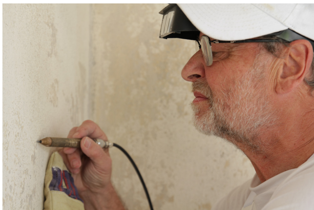
10 Mies van der Rohe and Lilly Reich, Tugendhat House, Brno, Czech Republic, 1929-30. Ivo Hammer cleaning of the original façade plaster using pneumatic micro chisel. © Dieter Reifarth, 2011.
