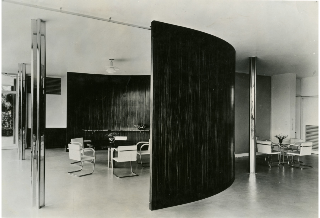
03 Mies van der Rohe and Lilly Reich, Tugendhat House, Brno, Czech Republic, 1929-30. Living room, semi-circular wall consisting of Macassar ebony veneer of the dining area. © Rudolf de Sandalo, 1931.
