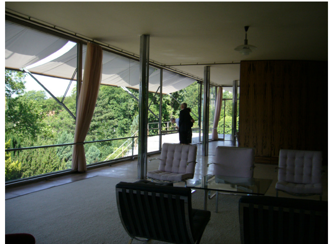
09 Mies van der Rohe and Lilly Reich, Tugendhat House, Brno, Czech Republic, 1929-30. Main living room, view towards west, before restoration: PVC flooring, semicircular wall not matching the original one, distemper paint on the ceiling, plastic curtains, commercial copies of the furniture. © Ana Tostões, 2009.
