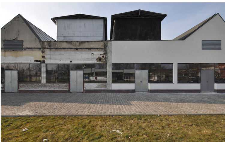
09 Mies van der Rohe, HE -building, Krefeld, Germany, 1930-1938. Dyeing plant façade, preserved state next to restored part. © Daniel Lohmann, 2016.
