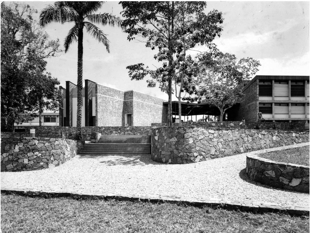
07 Michel Écochard, University of Yaoundé, Cameroon, 1963-1967, view of the main buildings. © Aga Khan Trust for Culture (AKTC).
