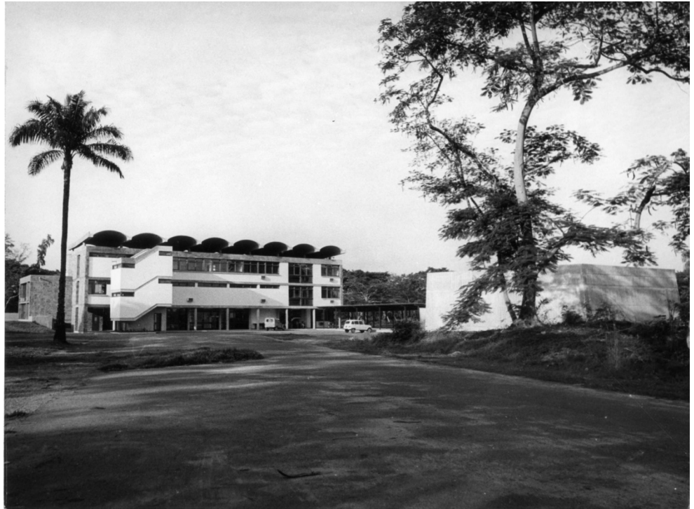
06 Michel Écochard, University of Congo, Brazzaville, 1963, Nain university building with concrete barrel vaults that function as a climatic roof that are offer monumental expression. © Aga Khan Trust for Culture (AKTC).
