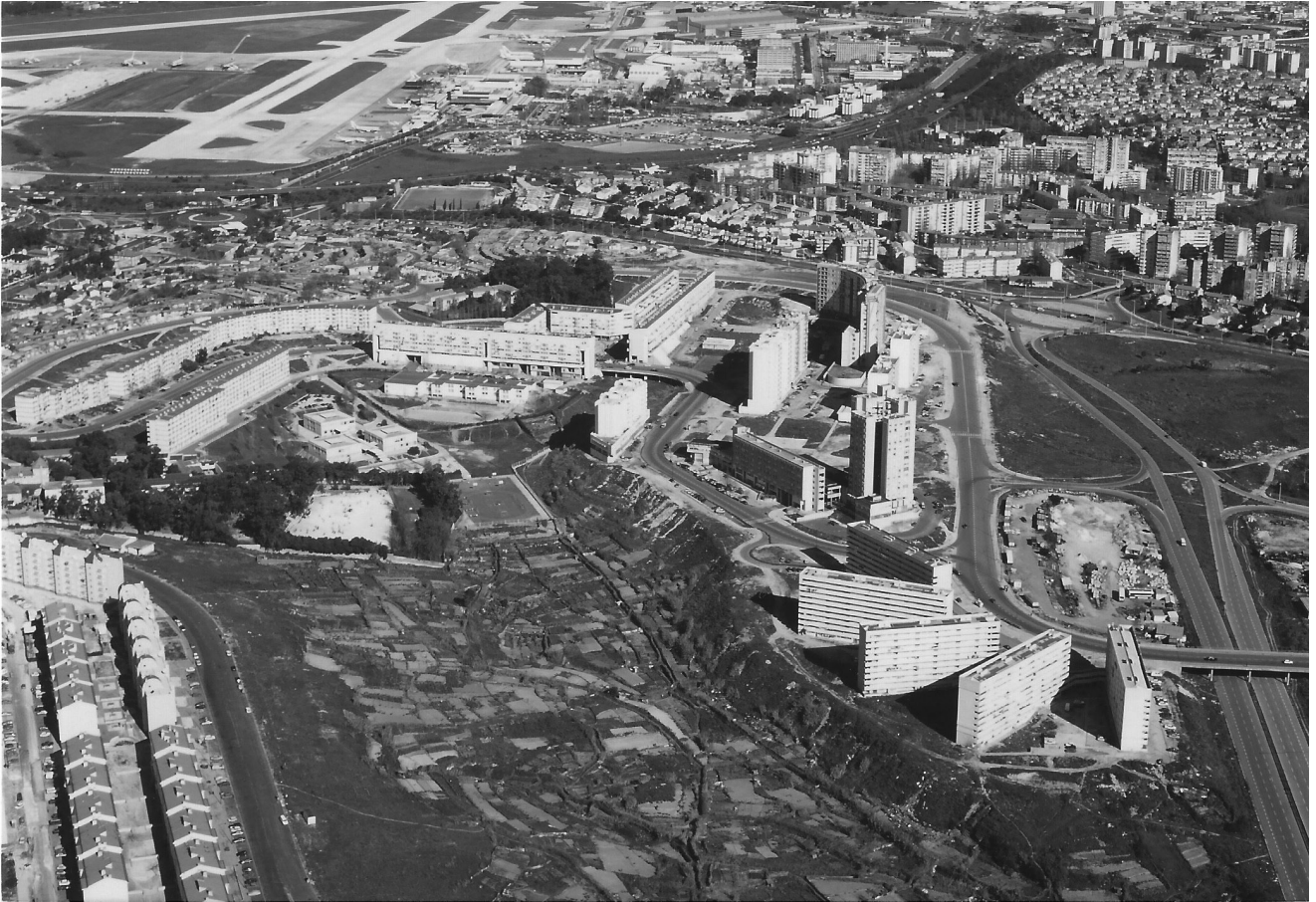
08 Aerial view of Cluster N2, Lisbon, Portugal. © José Luís de Brito, 1995.
