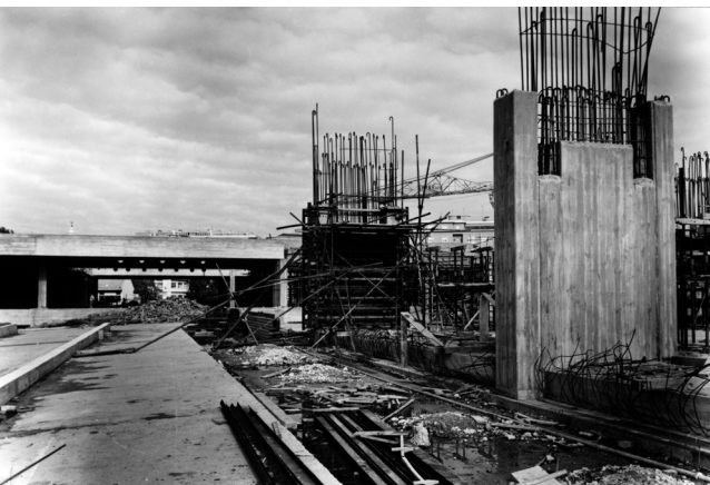
03 Alberto Pessoa, Pedro Cid, Ruy Jervis d'Athouguia, Calouste Gulbenkian Foundation, Lisbon, Portugal, 1959-1969, headquarters concrete pillars. © FCG Archive, 1965.
