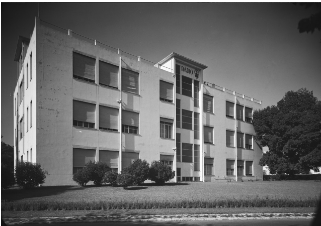
08 Carlos Ramos, Radium Pavilion, Portuguese Institute of Oncology, Lisbon, Portugal, 1933. Southeast façade. © Art Library of Calouste Gulbenkian Foundation [CFT003_125240].
