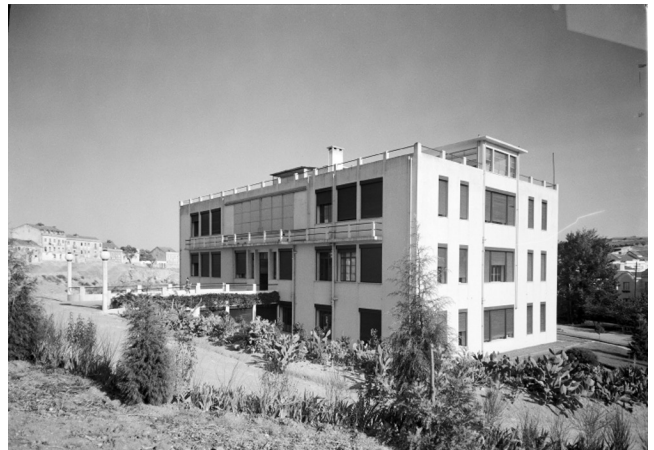
09 Carlos Ramos, Radium Pavilion, Portuguese Institute of Oncology, Lisbon, Portugal, 1933, Northwest façade © Art Library of Calouste Gulbenkian Foundation [CFT003_63485].
