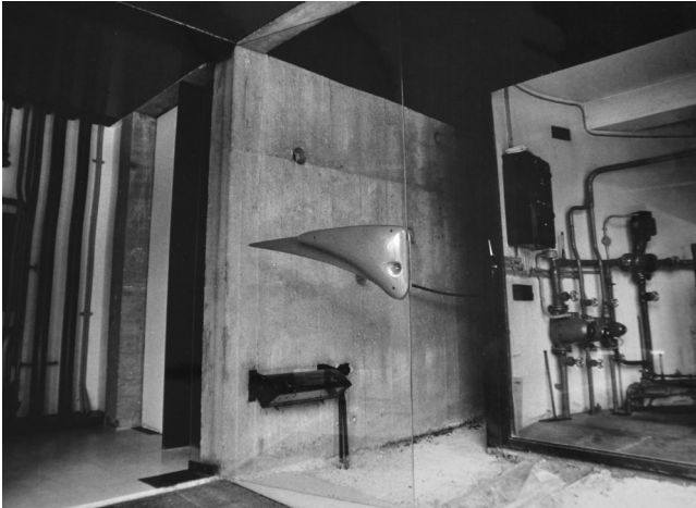
03 André Wogenscky and Marta Pan, House/Workshop, Saint-Rémy-lès-Chevreuse, France, 1950-1952. The entrance: Boiler and Marta Pan's door handle (Nowadays, the same model is visible). © Archives wsr, Fondation Marta Pan-André Wogenscky.
