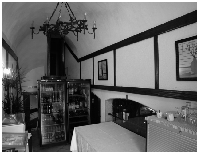
07 Alberto Sartoris, Cercle de l'Ermitage , Epesses, Switzerland, 1935. Gallery. Le Vieux Moulin, le Cercle de l'Ermitage disappears under a jumble of fake beams and stucco. © Jean-Christophe Dunant, 2010.
