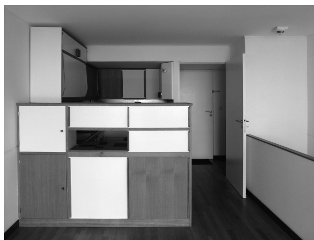
07 Le Corbusier, Unité d'Habitation , Marseille, France, 1945-1952. Reconstruction of fire-damaged apartments. A kitchen and its furniture fully rebuilt identically. © Photo F. Botton/ssea, September 2014. FLC/2016, Prolitteris, Zurich.
