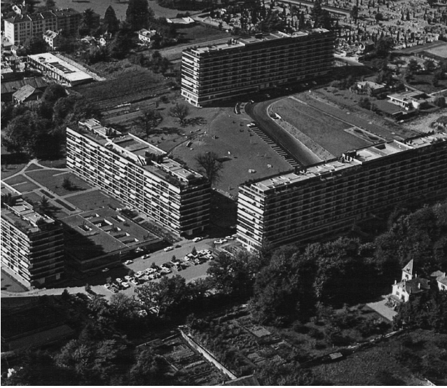
05 Georges Addor, Jean-Jacques Honegger, Budé Housing Estate, Geneva, 1958-1962. © Addor & Julliard Archives, Geneva.
