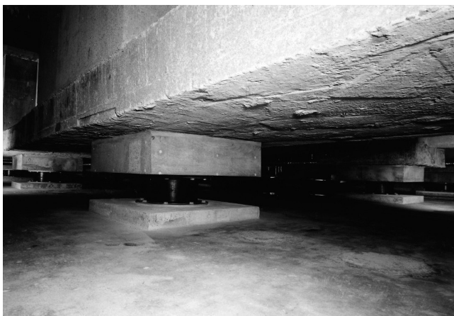
06 Le Corbusier, National Museum of Western Art, Tokyo, Japan, 1959. Seismic Isolation Retrofit © NMWA, 2007.
