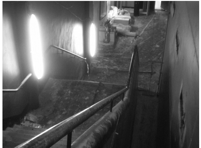
12 Le Corbusier and Pierre Jeanneret, Cité de Refuge , Paris, France, 1933. The staircase leading from the lobby to the large meeting room on the ground floor, protected by listing as a historical monument in 1975, was restored to its original form in February 2015. © Gilles Ragot, 2015.
