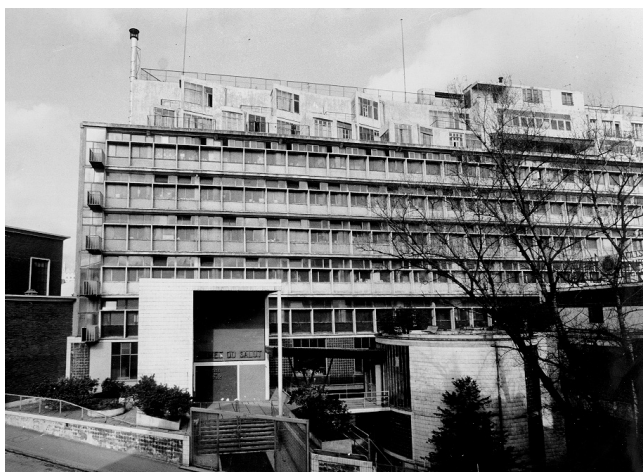
03 Le Corbusier and Pierre Jeanneret, Cité de Refuge , Paris, France, 1933. South façade in the early 1970s with a brise-soleil installed in 1952. The volumes of the two upper floors were to be restored in the construction works of 1973–1977. © L2-4-43-001 FLC/SPA.
