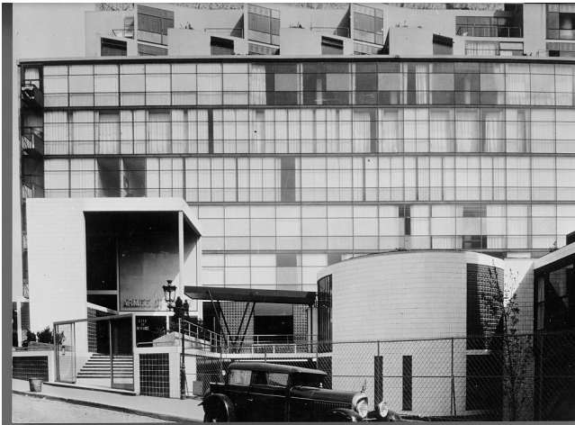
01 Le Corbusier and Pierre Jeanneret, Cité de Refuge , Paris, France, 1933. South Façade Glass Curtain Wall in 1933. © L2-4-41-001 FLC/SPA.
