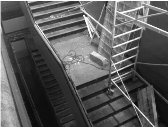
11 Le Corbusier and Pierre Jeanneret, Cité de Refuge , Paris, France, 1933. The staircases are opened to provide the original spatial fluidity. © Gilles Ragot, 2015.
