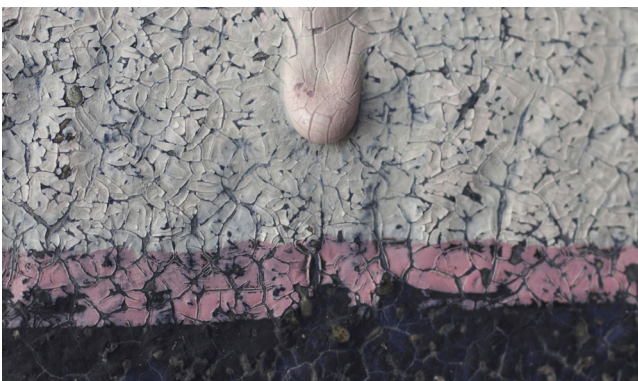
09 Le Corbusier, Detail of a drip mark and crazing, Coin Salle à Manger , Villa E-1027, Roquebrune-Cap-Martin, France. © Marie-Odile Hubert, 2011.
