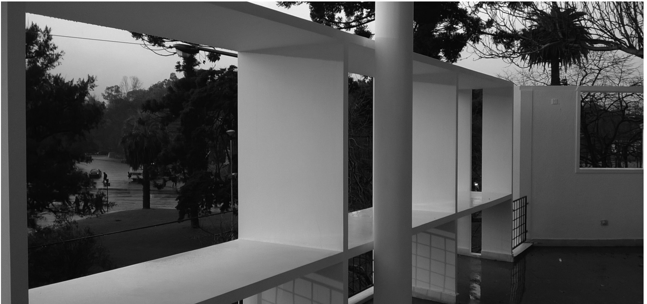
07 Le Corbusier, Maison Curutchet , La Plata, Argentina, 1949 - 1955. View to the park through the brise-soleil of the garden terrace. © Julio Santana, September 2014.
