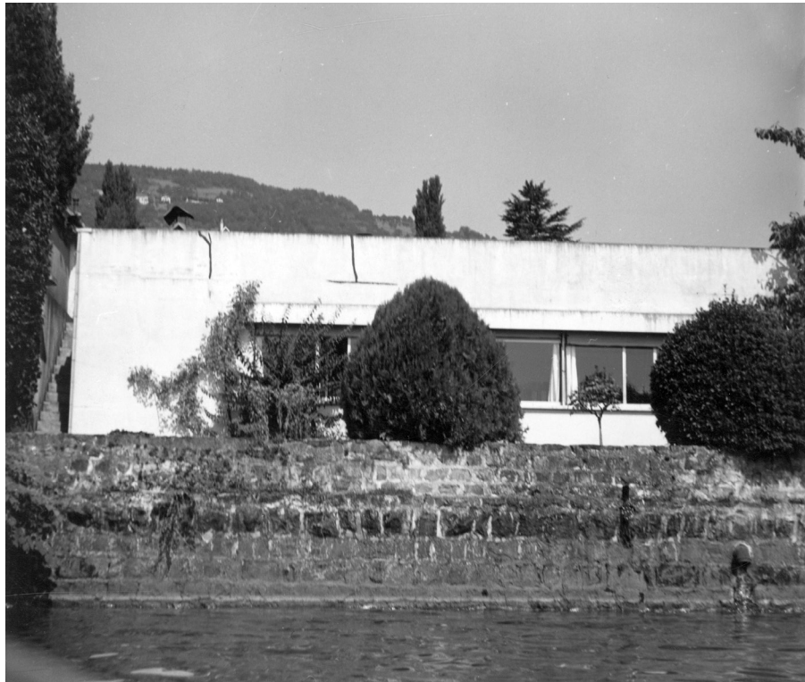
08 Le Corbusier and Pierre Jeanneret, Villa Le Lac , Corseaux-sous-Vevey, Switzerland, 1924, South façade with cracks, © FLC/SPA, between 1941 and 1951.
