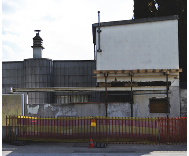
05 Le Corbusier and Pierre Jeanneret, Petite Maison , Corseaux, Switzerland, 1924. The original steel I-beam after restoration. © Giulia Marino, 2014.
