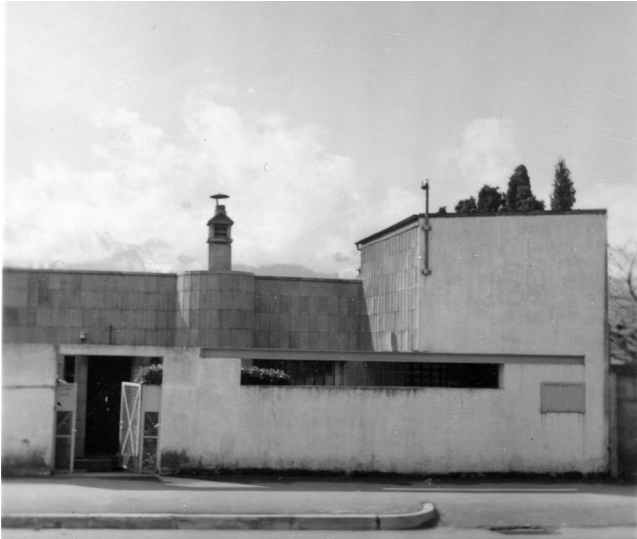
04 Le Corbusier and Pierre Jeanneret, Petite Maison , Corseaux, Switzerland, 1924. The wall that closes off the property on the north, a steel I-beam supporting the fruitière , 1924. © Le Corbusier, Une Petite Maison , Artemis, 1954.
