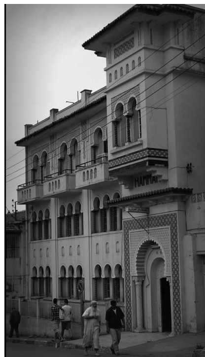
03 X. Salvador, DPIC., M. Garnier, Perret Brothers, Civil Hospital, Sétif, Algeria, 1935-1938. Engineering and execution Ch. Tisserand companies. © Chantiers, Archives of the Department of Algiers, 1938.
