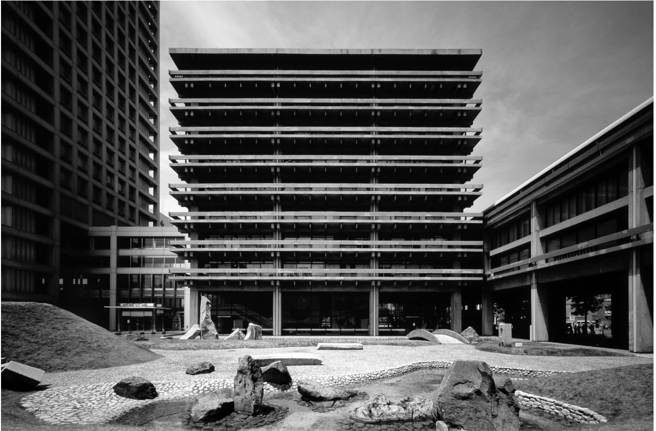
01 Kenzo Tange, The Kagawa Prefectural Government Office East building, Kagawa, Japan, 1958. Outer view of the East building which shows the expression of traditional Japanese wooden architectural ideas. © Toshihiro Misaki, 2009.
