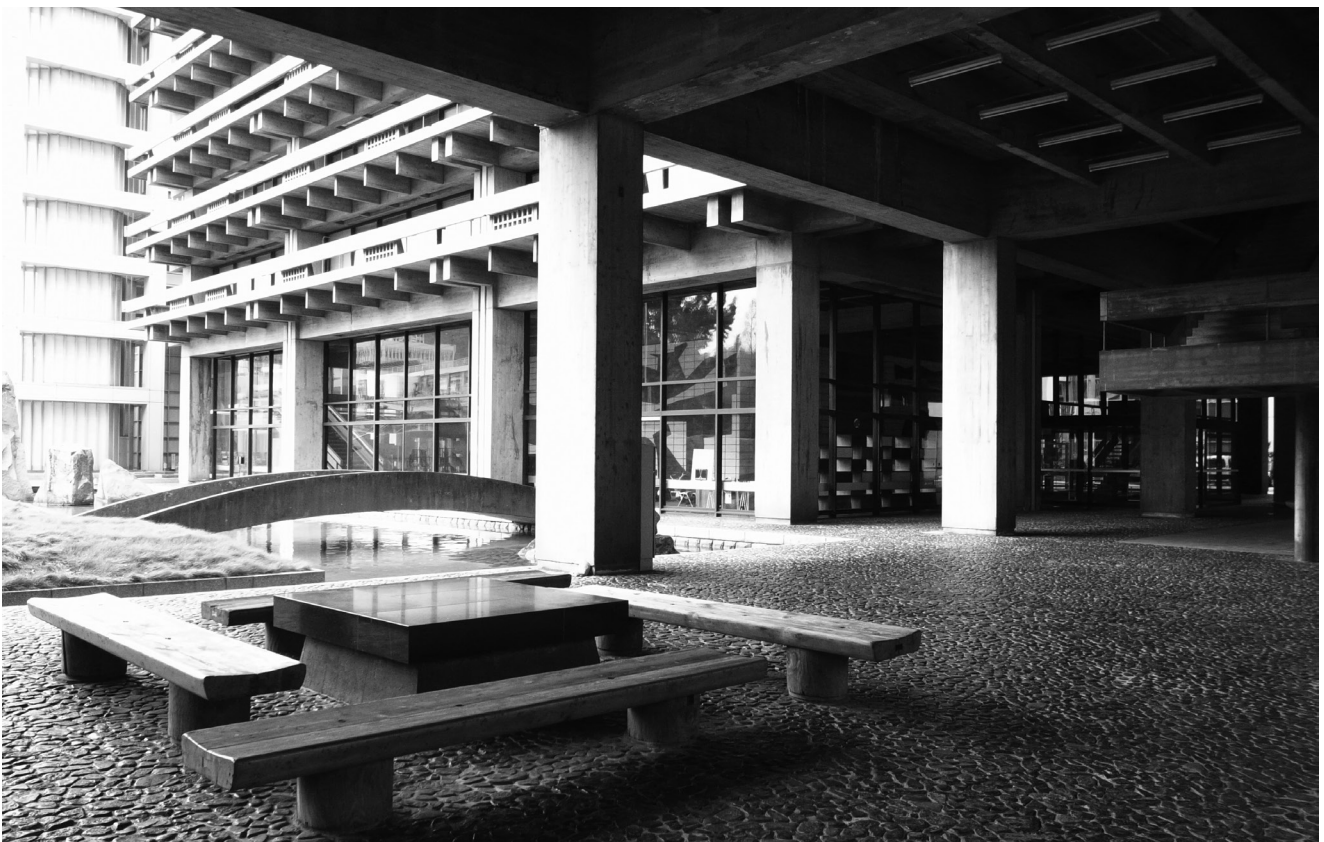
02 Kenzo Tange, The Kagawa Prefectural Government Office East building, Kagawa, Japan, 1958. The open-plan piloti which connect the lobby and the south garden. © Kagawa Prefecture, 2014.
