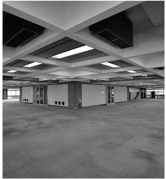
05 Kenzo Tange, The Kagawa Prefectural Government Office East building, Kagawa, Japan, 1958. An open office space. © Seiji Izumi, 2014.
