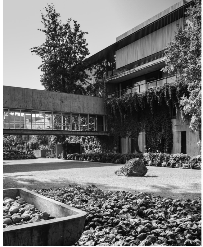
13 Emilio Dubart, ECLAC building, Santiago, Chile, 1966. Reuse design by O1ARQ, Pablo Saric, Cristian Winckler, Felipe Fritz, 2011. New Pavilion, view from the north-west patio. © Aryeh Kornfeld, 2013.
