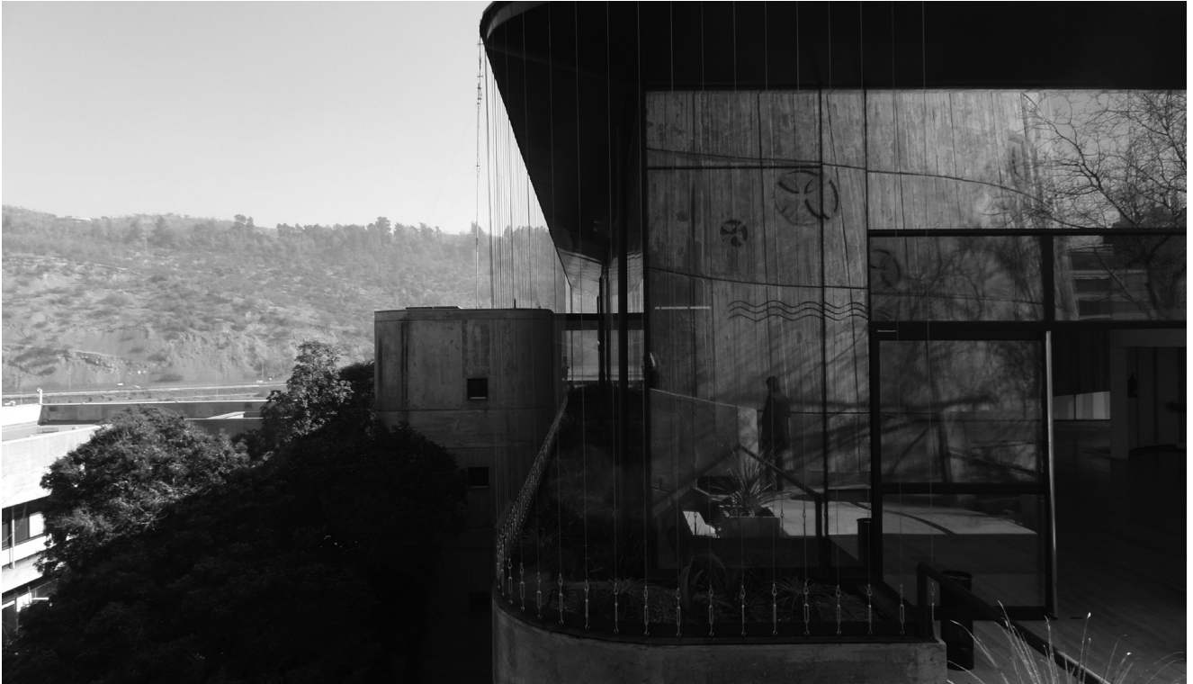
15 Emilio Dubart, ECLAC building, Santiago, Chile, 1966. Reuse design by O1ARQ, Pablo Saric, Cristian Winckler, Felipe Fritz, 2011. New Pavilion, view from the stairs of the Caracol . © Horacio Torrent, 2014.
