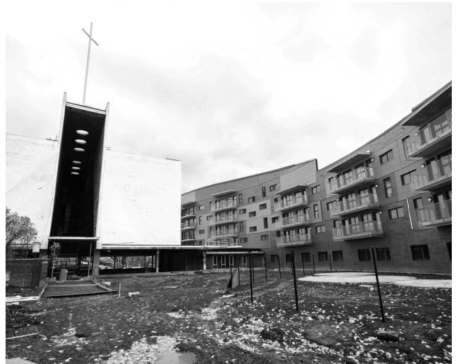
05 Gérard Notebaert, Church Sainte-Germaine-Cousin , Montreal, 1960-1962 and Rayside Labossière Architectes, Sainte-Germaine-Cousin dwellings, Montreal, 2005-2014. Outside view of the building site as the new building is almost completed. © Saul Rosales, Rayside Labossière Architectes, 2014.
